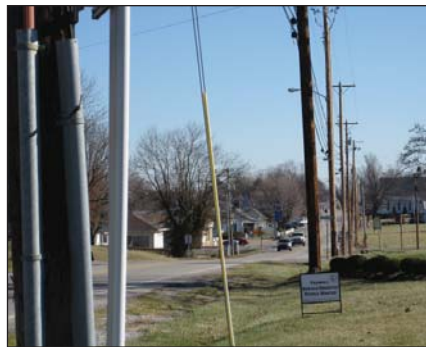
No sidewalk, overhead utilities
