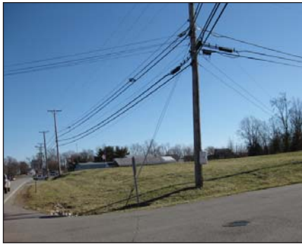
Overhead utilities, vacant lot, no sidewalk or crosswalk
