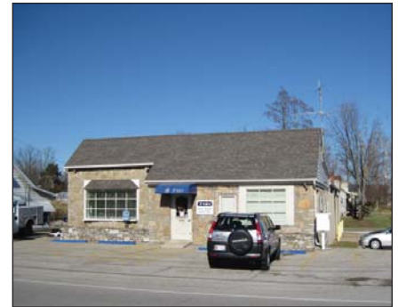
Unrestricted access, building setback used as parking
