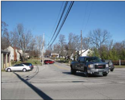
No definition between roadway and property line, overhead utilities
