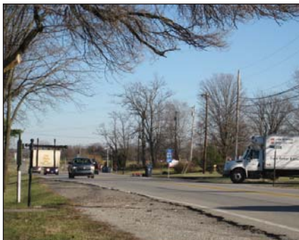
US 60 corridor (looking east)
