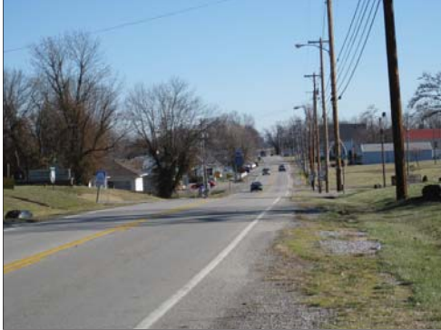
US 60 corridor (looking east)
