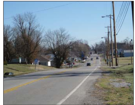
US 60 corridor (looking east)
