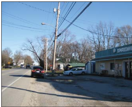
Unrestricted access, outdoor storage, overhead utilities
