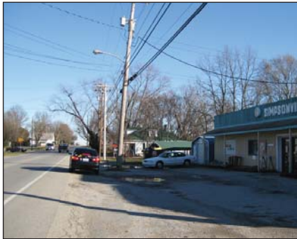
Unrestricted access, outdoor storage, overhead utilities
