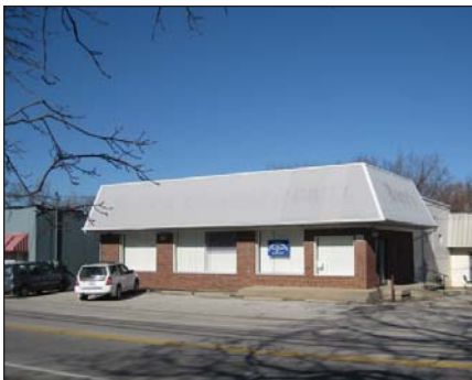
Unrestricted access, setback used as parking
