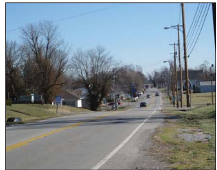
US 60 corridor (looking east)
